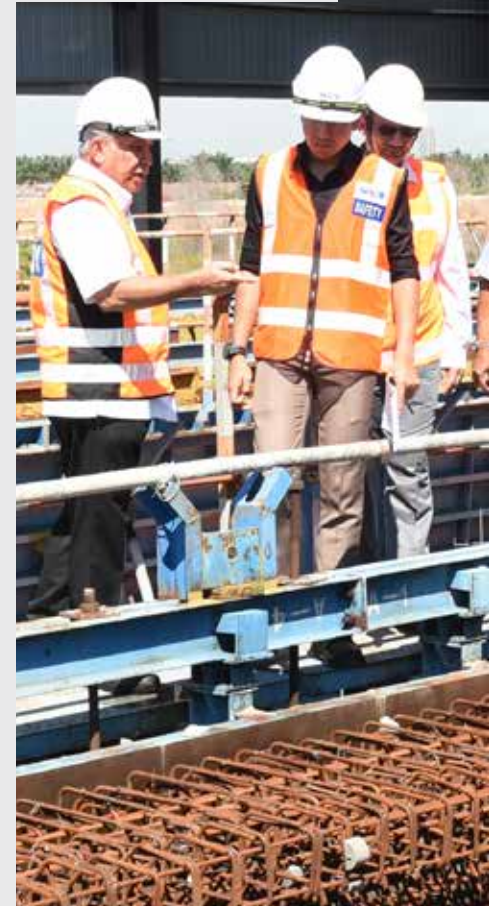
ODS working at a construction site
